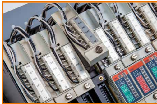
Reattach existing Field Wiring adaptors
