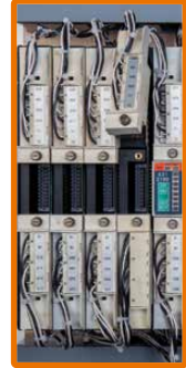
Replace controller card with Weidmuller adaptor card
